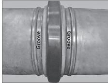
**4. JOIN PIPE ENDS:** Align and bring the two pipe ends together. Slide the gasket into position and center it between the grooves, as shown. Make sure no portion of the gasket extends into the groove in either pipe end.
