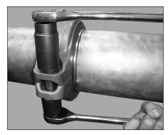
7. TIGHTEN NUTS: Tighten the nuts evenly by alternating sides. Make sure the housings' keys engage the grooves completely and the gaps are equal at the bolt pads. NOTE: It is important to tighten the nuts evenly to prevent gasket
