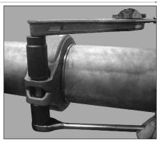
8. APPLY TORQUE: Apply torque to each nut with a torque wrench. Refer to the "Style D08 Torque Requirements" table below.
