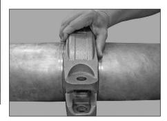
**5. INSTALL HOUSINGS:** Install the housings over the gasket with the tongue and recess features mated properly (tongue in recess). Make sure the housings' keys engage the grooves completely on both pipe ends.
